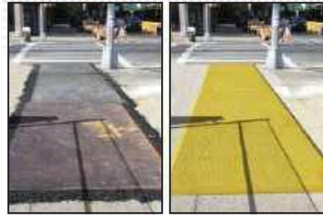
Steel Plates with Cold Patch
